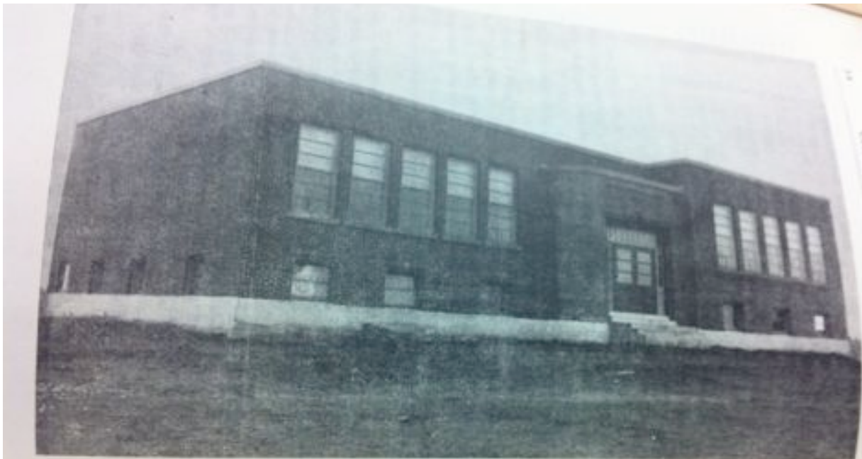
A New Four Classroom School
