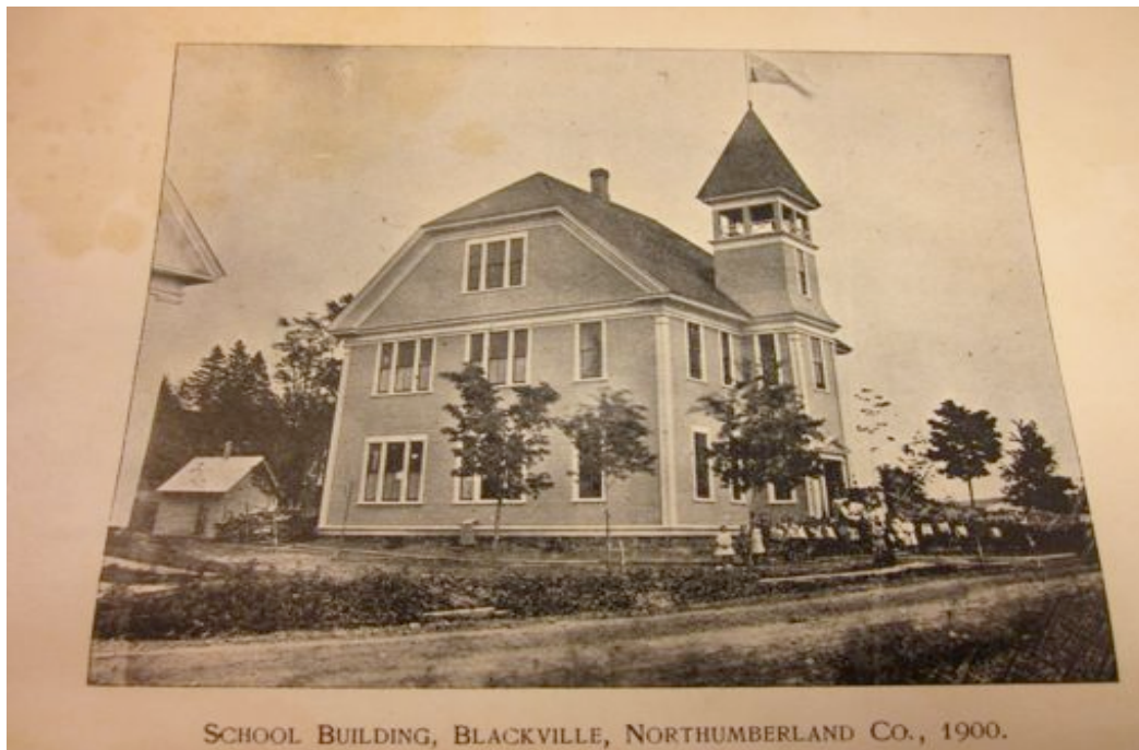
Fig. k. Image of School Building in Blackville, NB circa 1900. 35
